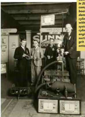
Sunnen is celebrating 90 years in 2014. This is a look at the company's old trade show booth, which often included demonstrations of the portable cylinder grinder (cylinder hone) with grit removal suction system. This allowed engine cylinders to be honed with the engine still in the chassis. The suction system removed the grit before it could fall down onto engine components.
